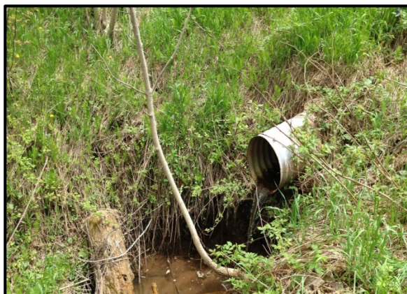
Perched outlet of culvert conveying Tributary E, downstream (north) of Sideroad 26/27 (May 22, 2014).
