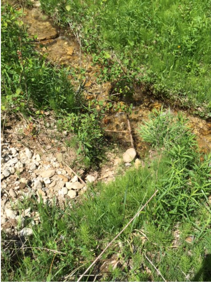
Photo 2 - Road material entering channel
