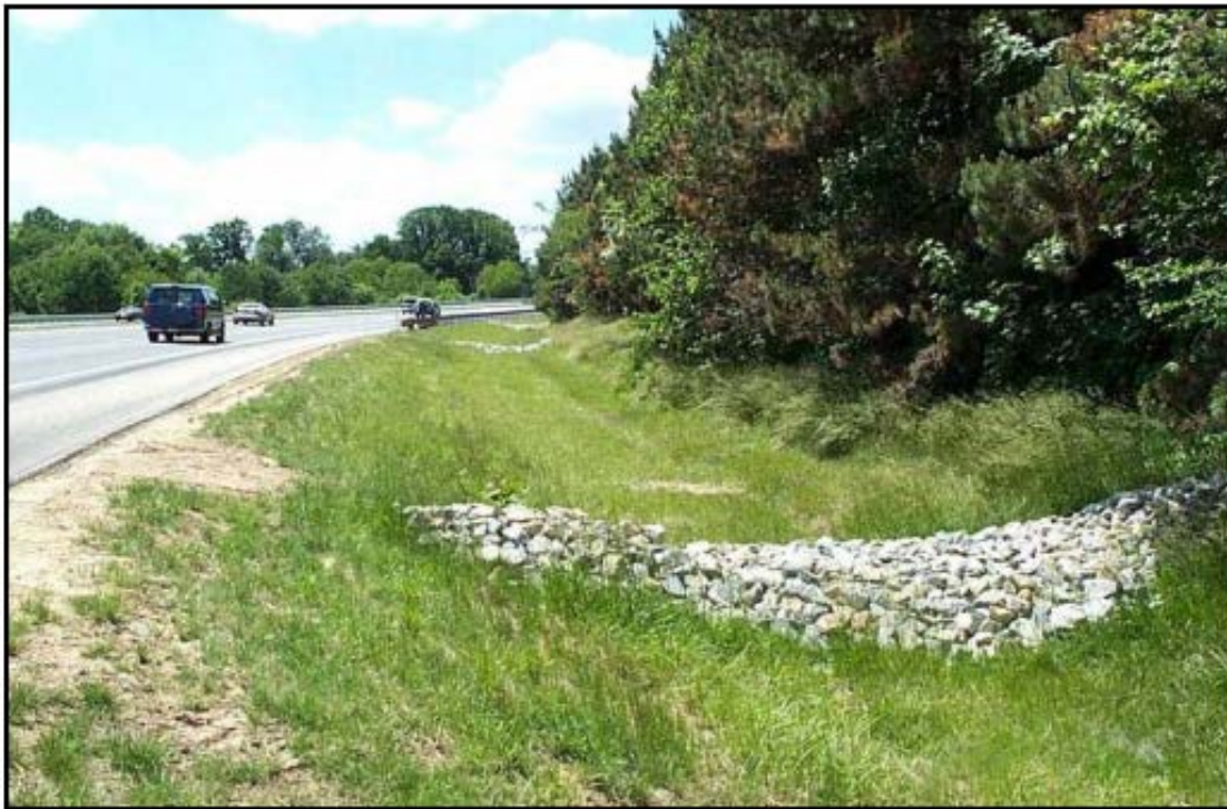
Figure 4.8.2 Enhanced grass swales feature check dams that temporarily pond runoff to increase pollutant retention and infiltration and decrease flow velocity
