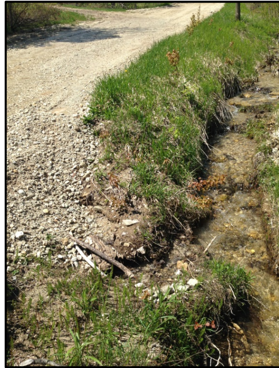
Road washout contributing coarse aggregate material to Reach 3 of Tributary A (April 27, 2015).
