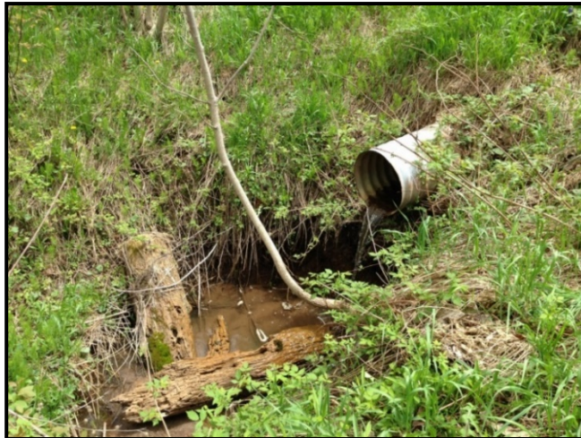
Photo 4: Perched outlet of culvert conveying Tributary E, downstream (north) of 26/27 Side Road (May 22, 2014)
